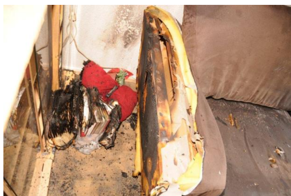
Foto 9: Secondaire brand woning 1 e verdieping
